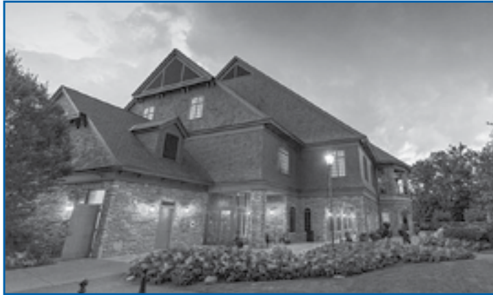
TURNING STONE CASINO SHENANDOAH CLUBHOUSE
